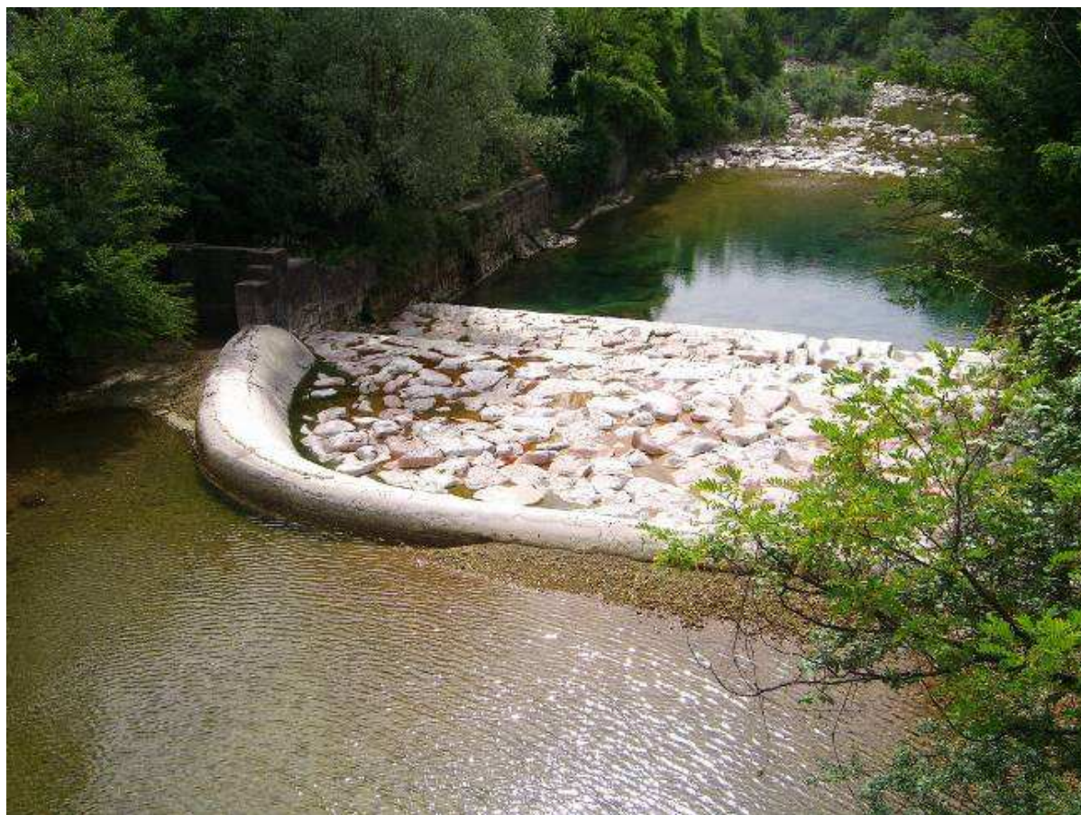
Figure 4: Measuring station at Ponte Pilo.
